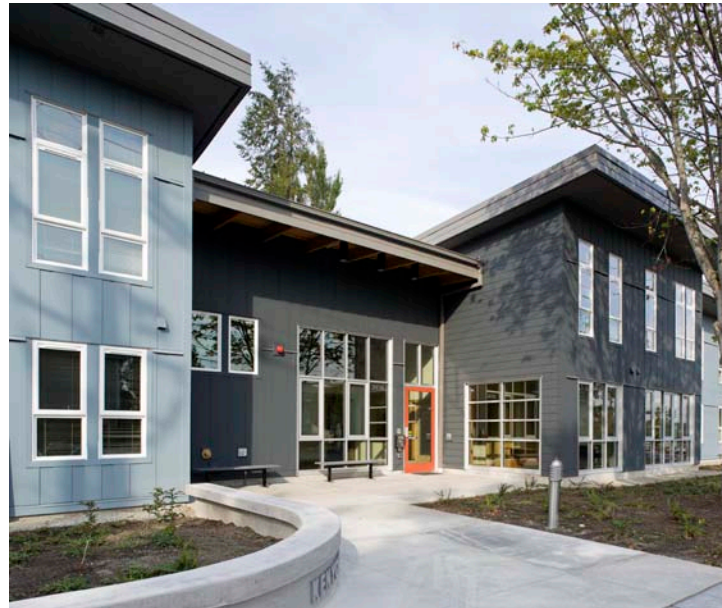
KENYON HOUSE 3936 S. Kenyon St. · Seattle Bellwether Housing/Building Changes
