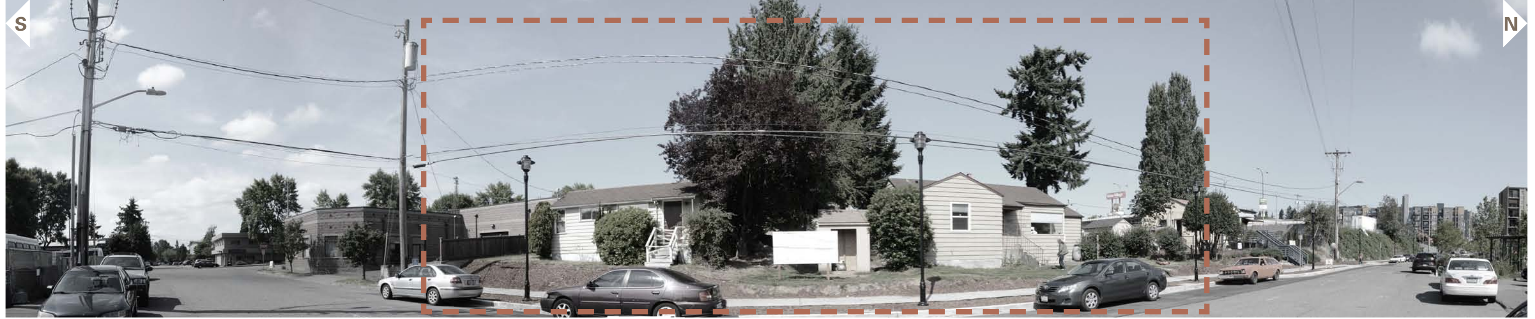
STREET ELEVATION- 33RD AVE. NE, EAST SIDE OF STREET
