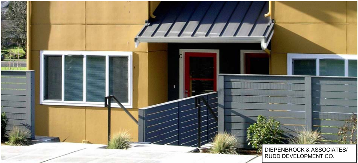
CEMENT PANEL WITH FLASHING REVEAL
