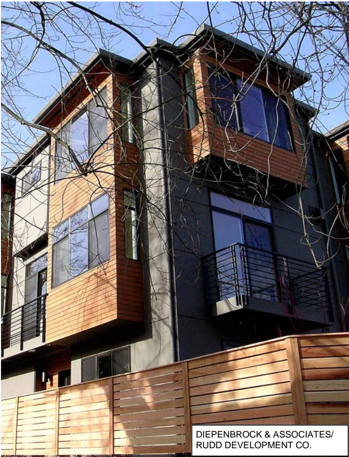
CEMENT PANEL WITH FLASHING REVEAL
