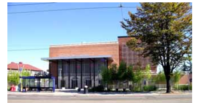
LINK LIGHT RAIL STATION
