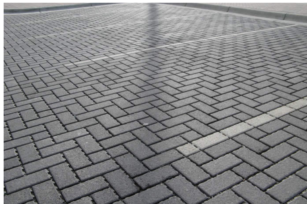
2. Permeable paving in the Right of Way
