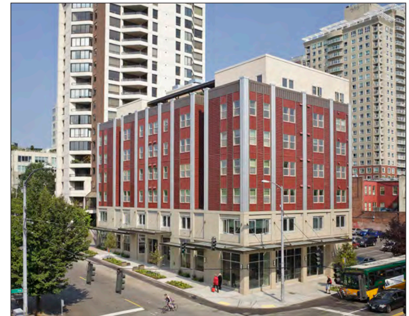
AL HUMPHREY HOUSE 2630 First Avenue Seattle, WA Plymouth Housing Group
