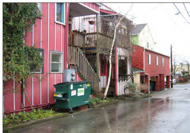
LOOKING NORTHWEST FROM ALLEY
