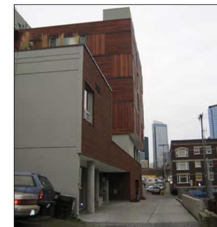
LOOKING SOUTH FROM ALLEY
