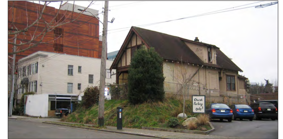
PROJECT SITE FROM NORTHEAST
