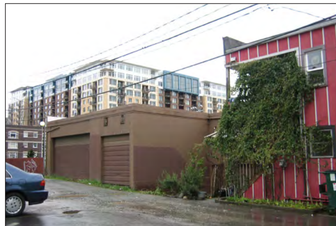
LOOKING SOUTHWEST FROM ALLEY
