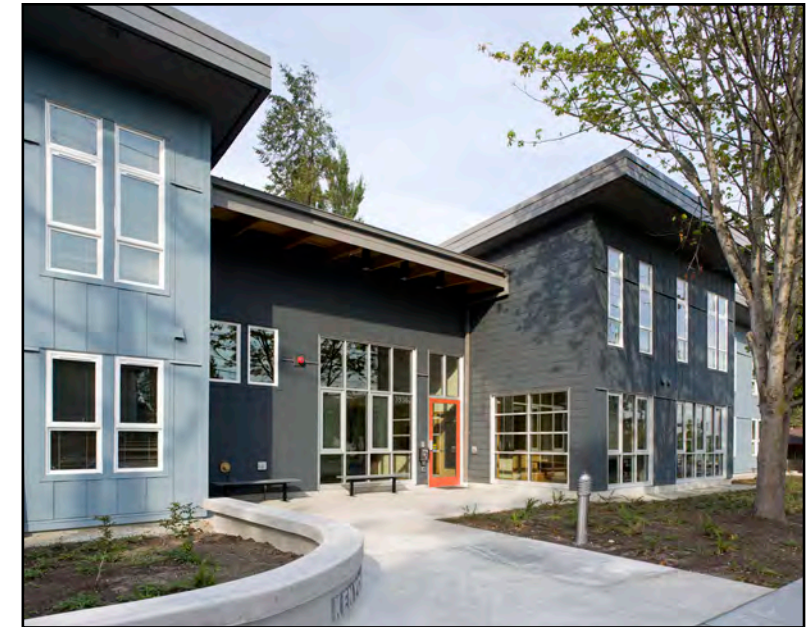
KENYON HOUSE 3936 South Kenyon Street Seattle, WA HRG
