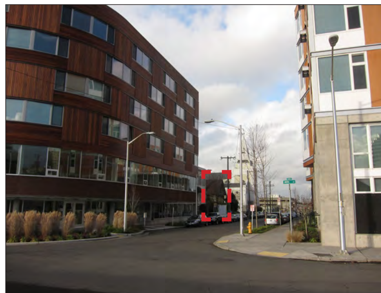
LOOKING NORTH ALONG PONTIUS AVENUE NORTH FROM JOHN STREET
