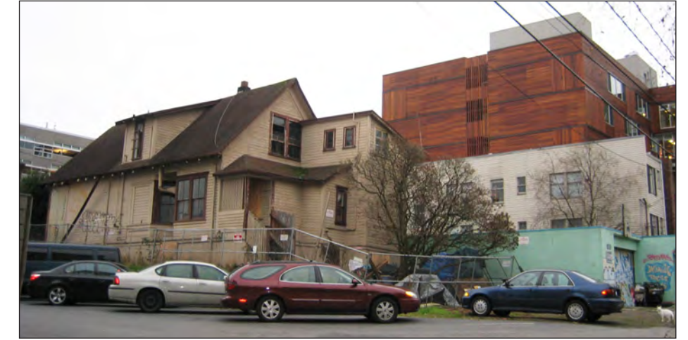
PROJECT SITE FROM NORTHWEST
