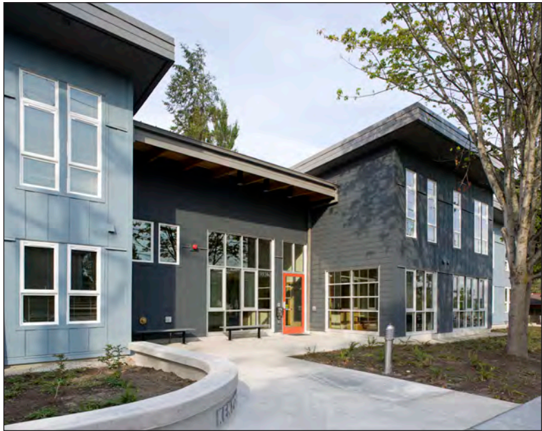
KENYON HOUSE for HRG: 3936 S. Kenyon St. On this building, fiber cement panels and siding are detailed in a clean, modern manner. The fascia is thick and strong, giving the masses an appropriate termination at the sky. Like Block 43, the project saved several large trees, which affected the design.
