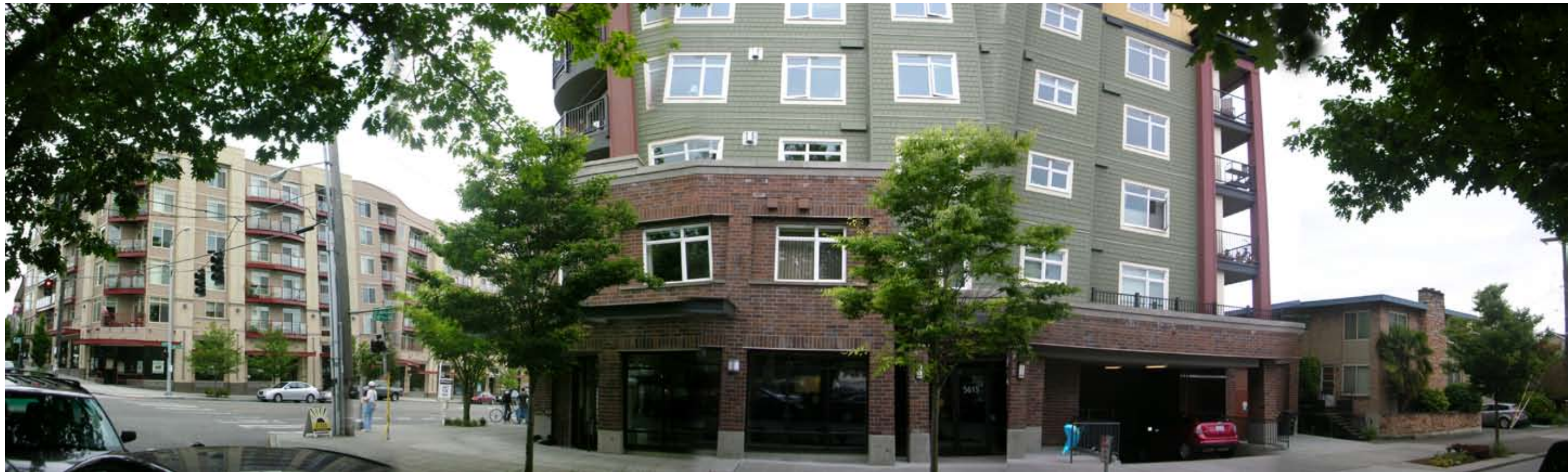
View South at 57th
