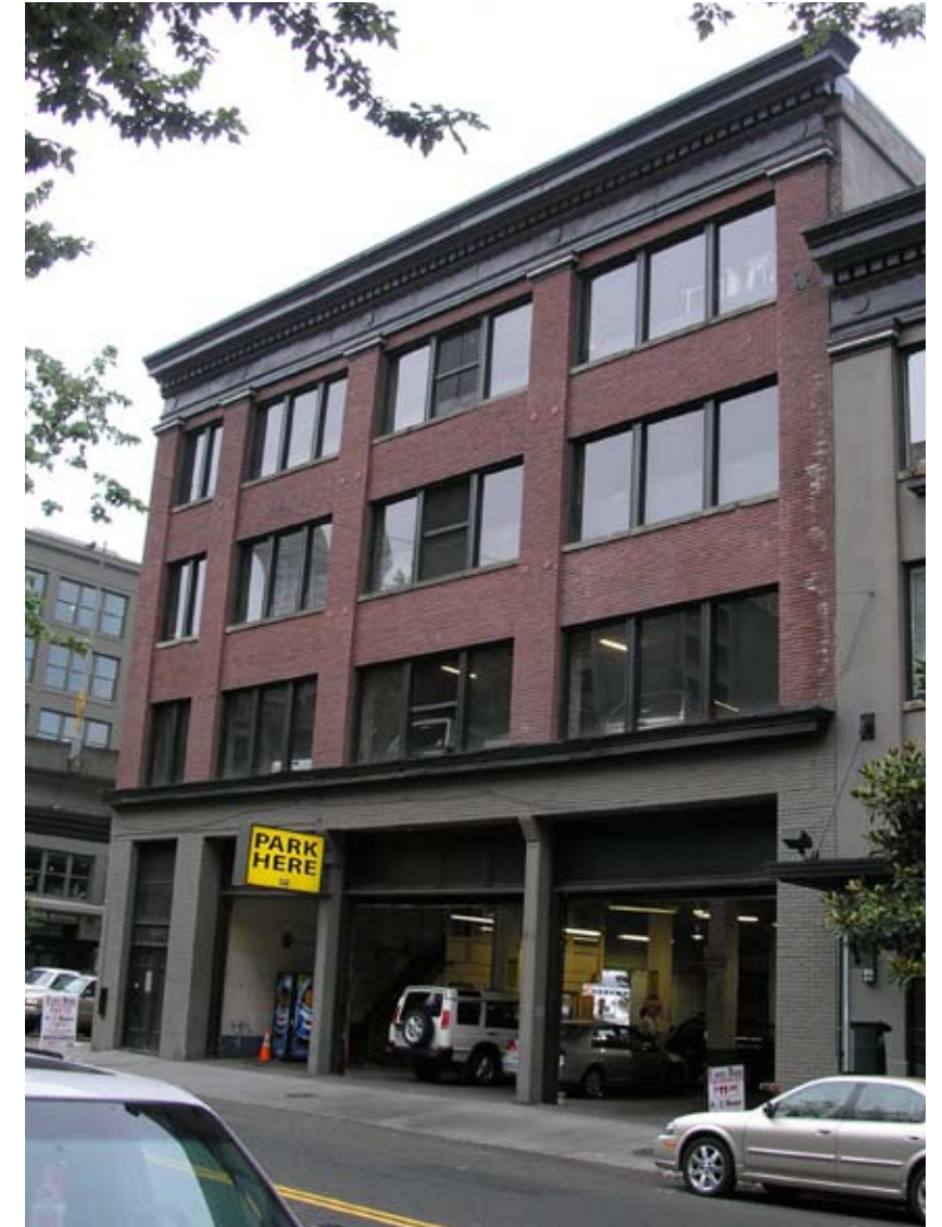
GARAGE ACCESS ON WESTERN
