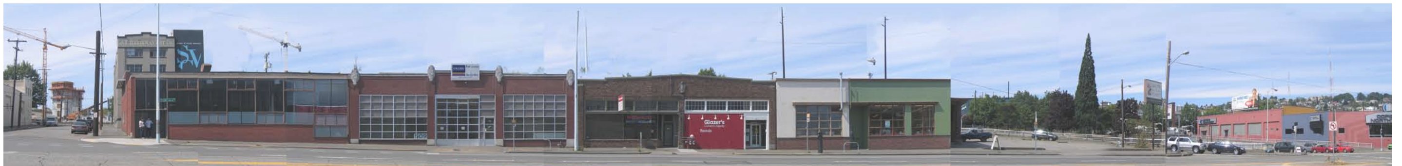
Adjacent Streetscape 4 - Dexter Avenue N (facing west)
