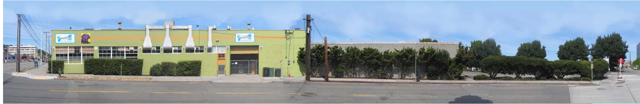
Site Elevation 1 - Republican Street (facing north)
