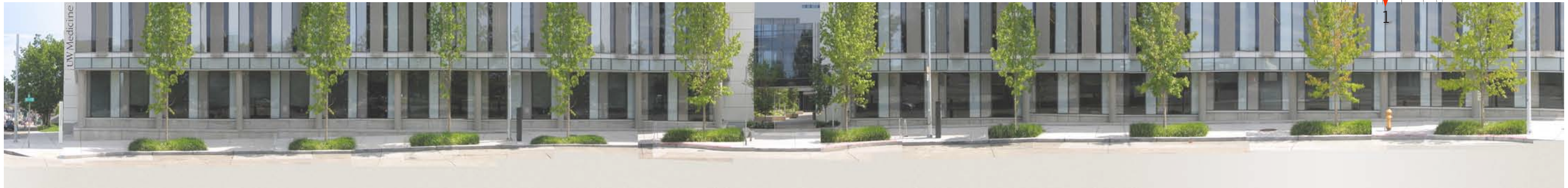
Adjacent Streetscape 2 - 8th Avenue N (facing east)
