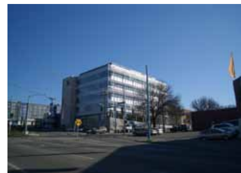
3 Fairview Research Center
