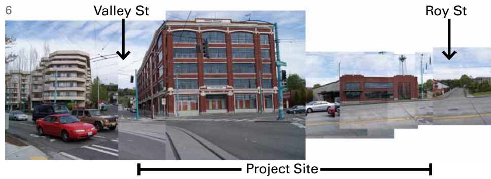
Fairview Avenue N - Looking East
