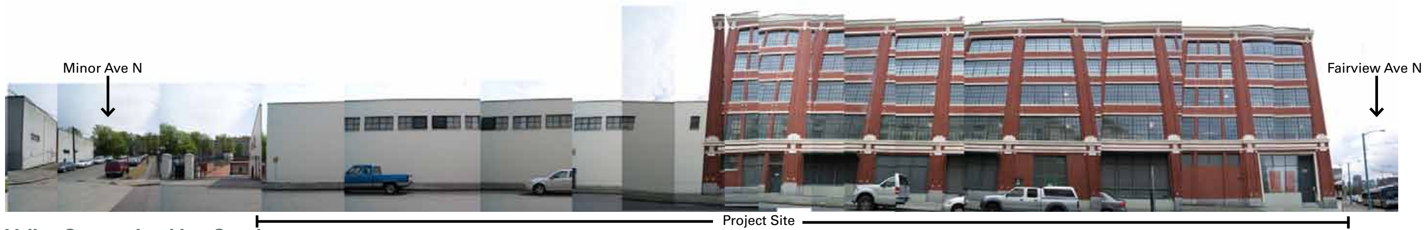
Valley Street - Looking South
