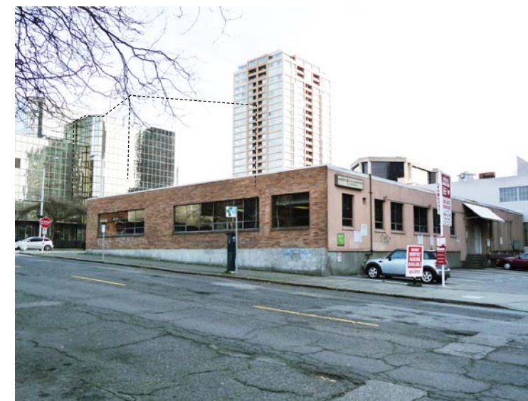
2 - Project Site looking SouthEast
