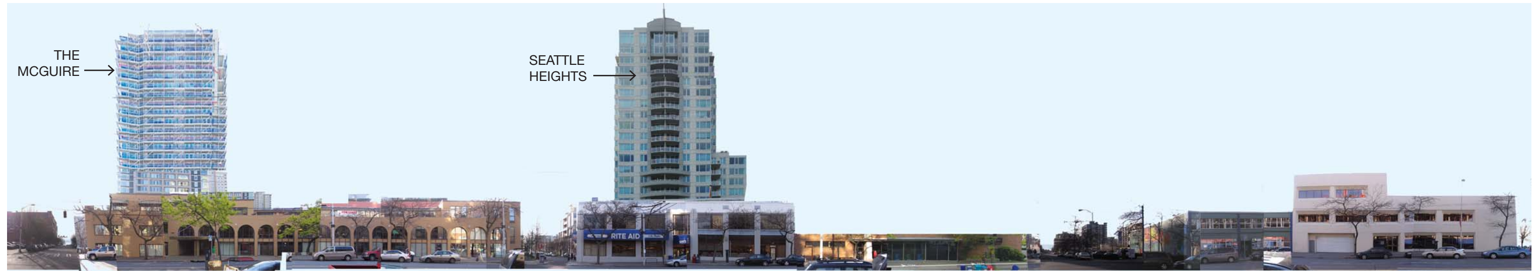
THE WEST SIDE OF 3RD AVENUE Vine Street Project Site Cedar Street
