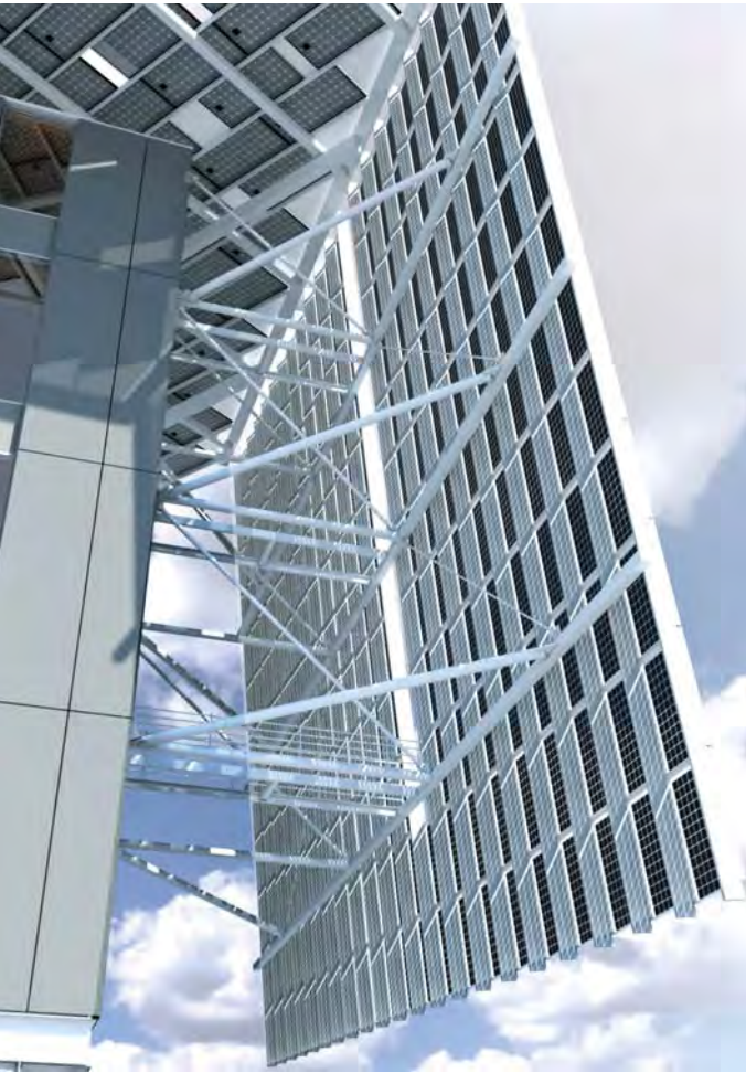
Close-up of vertical and rooftop PV arrays.
