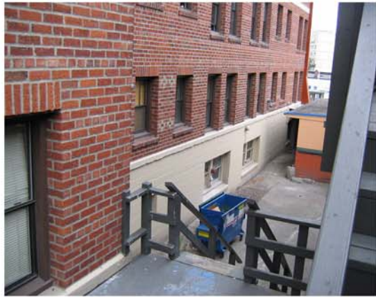
③ Existing Concrete Platform looking South
