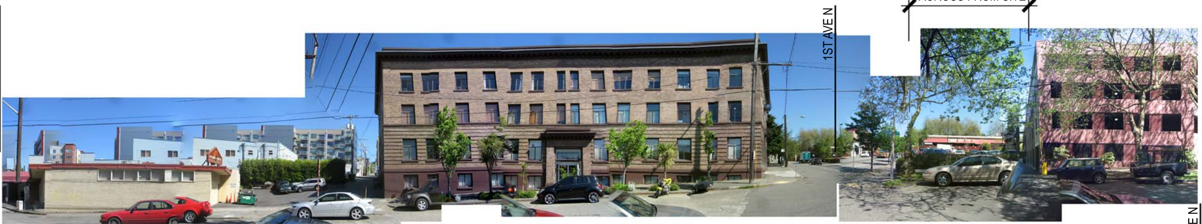
③ Street view along John Street, looking North
