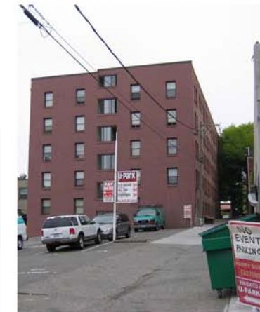
⑦ Southeast Corner - Alley
