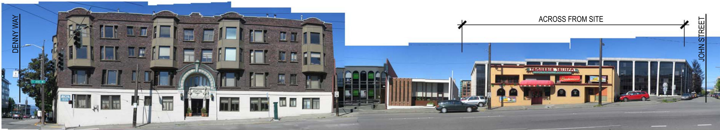
③ Street view along 1st Avenue North, looking West
