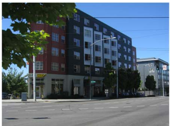
② Belltown Condominiums
