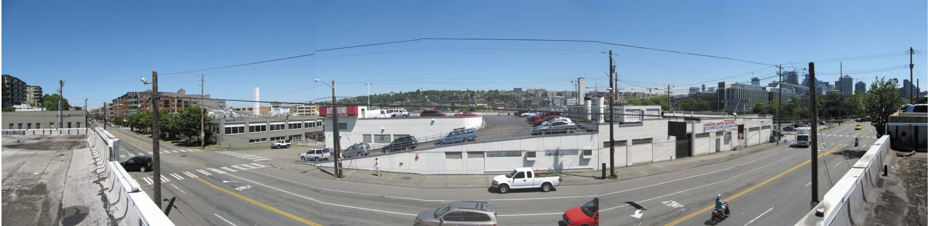
VIEW FROM PROPOSED LEVEL 3 LOOKING EAST
