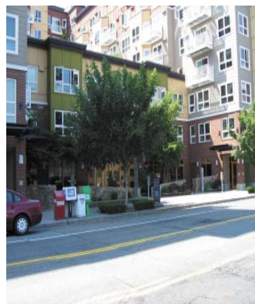
COURTYARD AT RES. ENTRY
