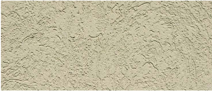
ELASTOMERIC PAINT ON STUCCO COLOR: GREENBRIER BEIGE / PARKER PAINT # HC-79 LOCATION: WALLS AROUND WARREN AVE. ENTRY
