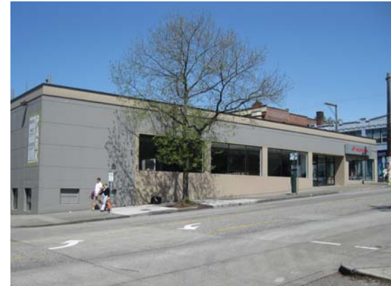
3 – Parking Garage / Vacant Storefront
