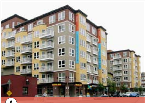
A 1200 Dexter Building - Apartments
