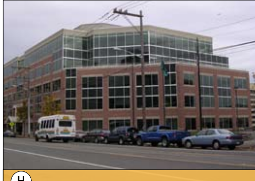
H 1000 Dexter - Office Building
