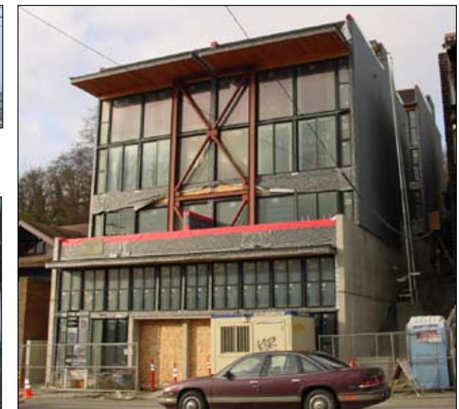
Multifamily building, Dexter Ave N, Seattle
