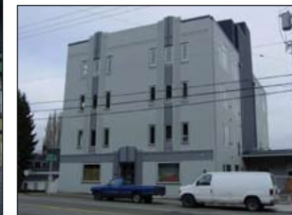
Multifamily building, Dexter Ave N, Seattle
