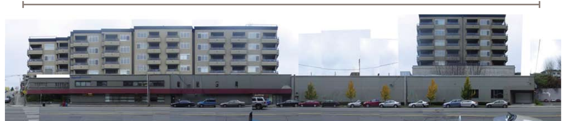
Dexter Ave. N - Looking W (toward site)
