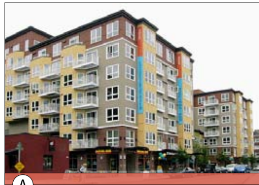
A 1200 Dexter Building - Apartments
