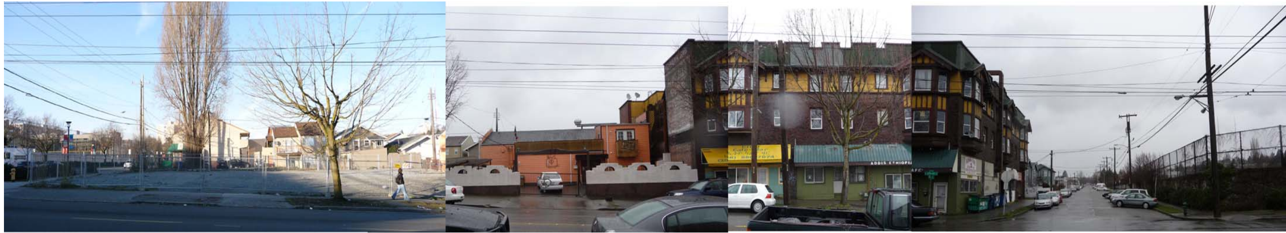
500 12th Avenue - Project Site
