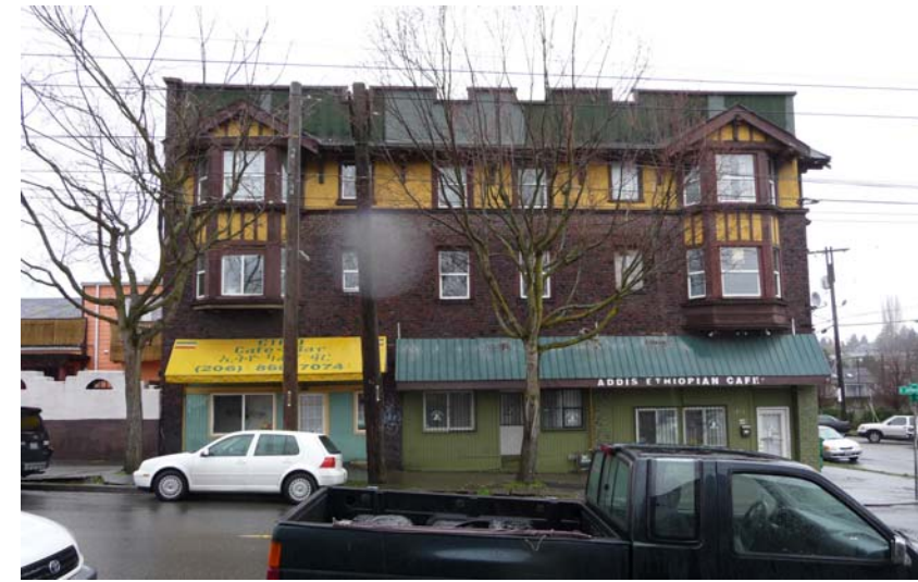
'Old' Mixed use building, East of Project site on the corner of E. Jefferson St. and 13th Ave S.
