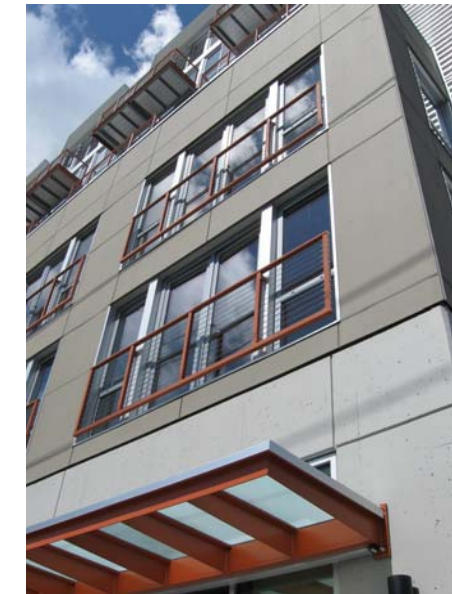
Siding and Balconies
