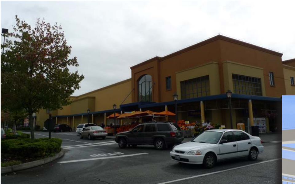
EXISTING PARKING LOT
