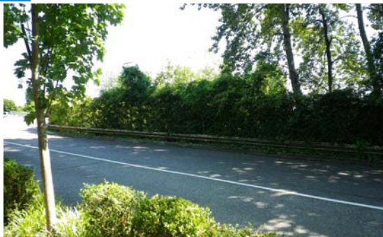
F Parking Lot Access Road
