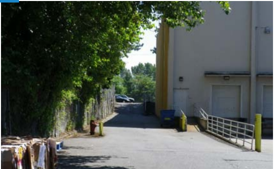
K Loading Dock Access
