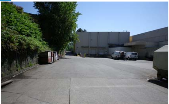
J Loading Dock Area
