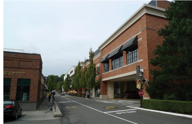
G Parking Garage
