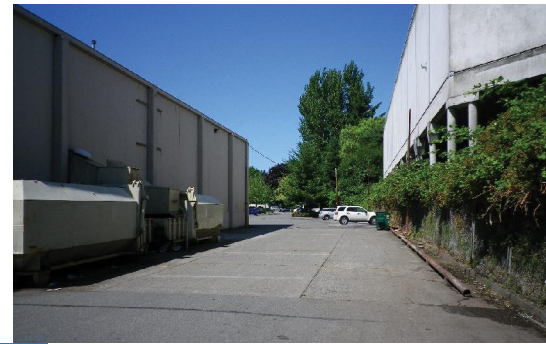
I Loading Dock Area
