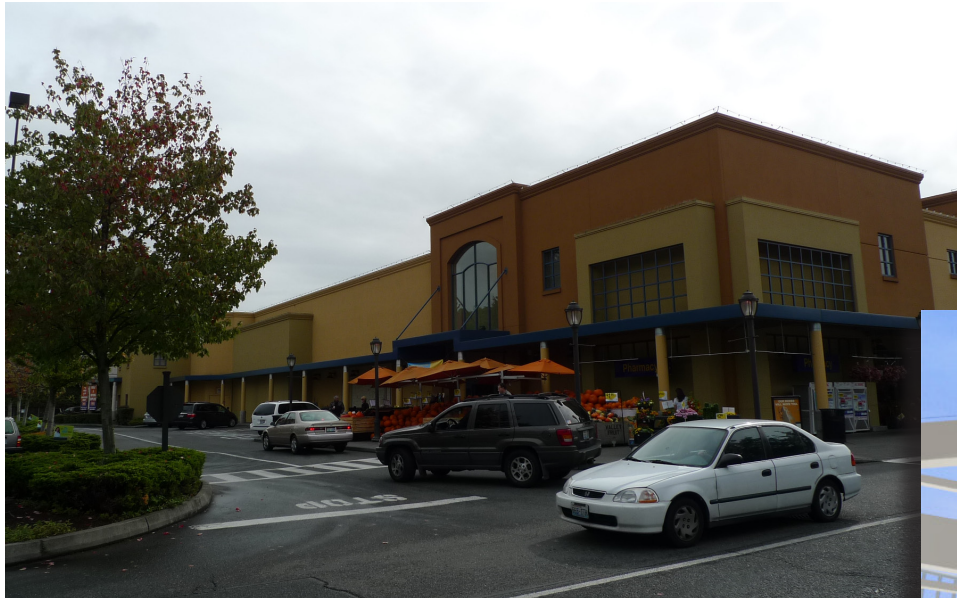
EXISTING PARKING LOT
