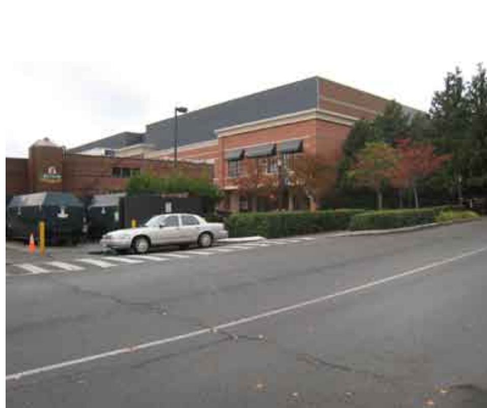
2 - Northwest Corner - Looking Northwest
