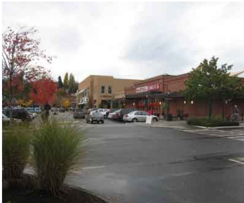
4 - Western Edge of Site - Looking Northwest
