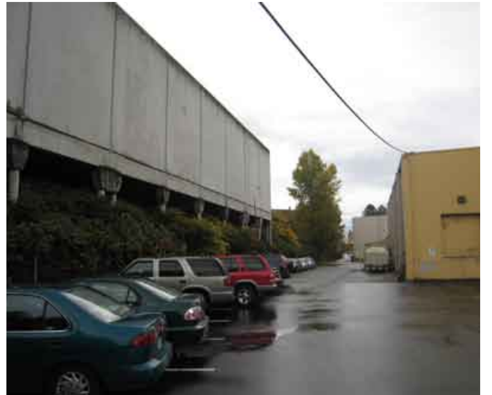
12 - Eastern Edge of Site - Looking South
