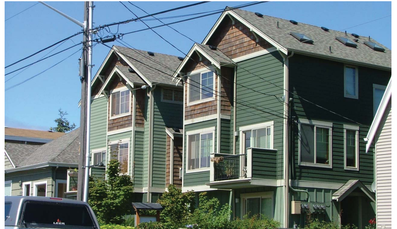
SITE PHOTO: VIEW OF MULTI-FAMILY PROJECT ON NW 63ND AVE WEST OF SITE
