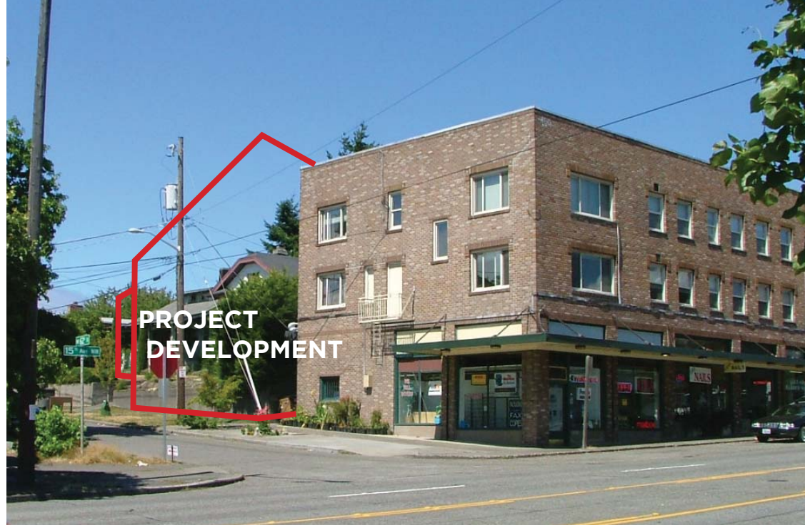
SITE PHOTO: CORNER OF 15TH AVE AND NW 62ND STREET
