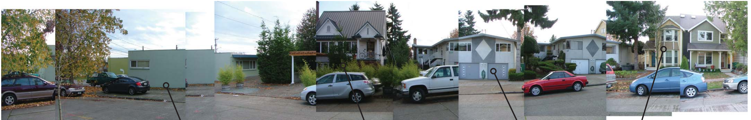
COMMERCIAL SPACE CMU and Concrete building
