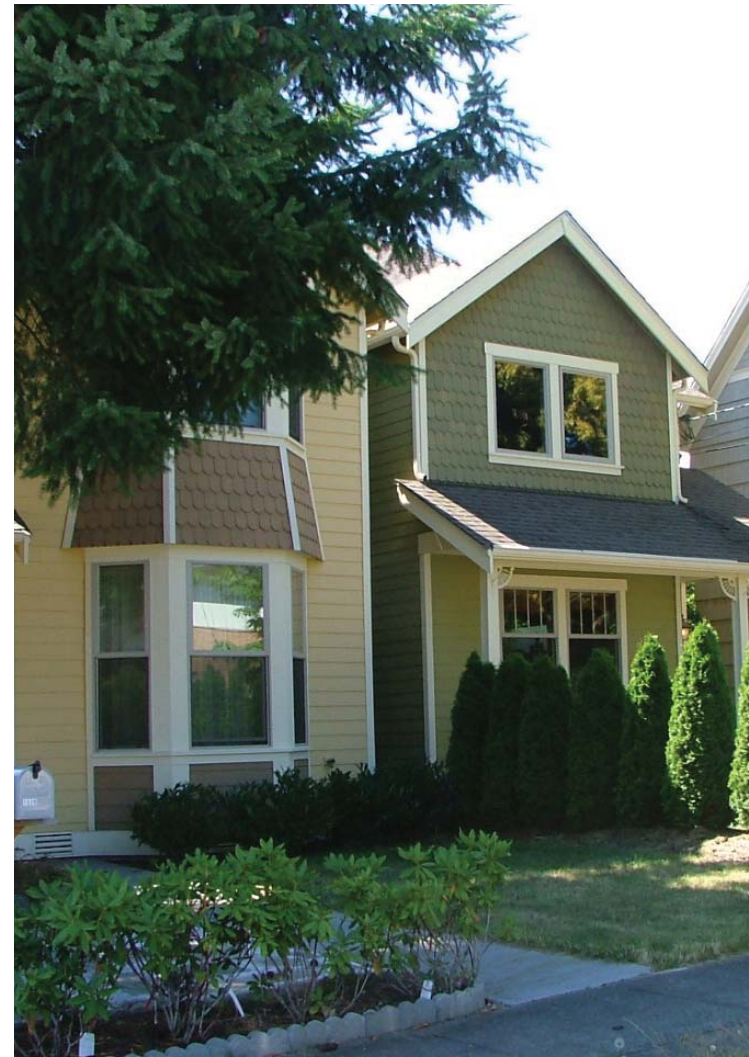
SITE PHOTO: VIEW OF MULTI-FAMILY PROJECT ON NW 62ND AVE WEST OF THE SOUTH
