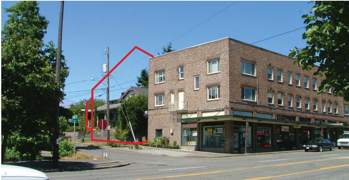
SITE PHOTO: CORNER OF 15TH AVE AND NW 62ND STREET
