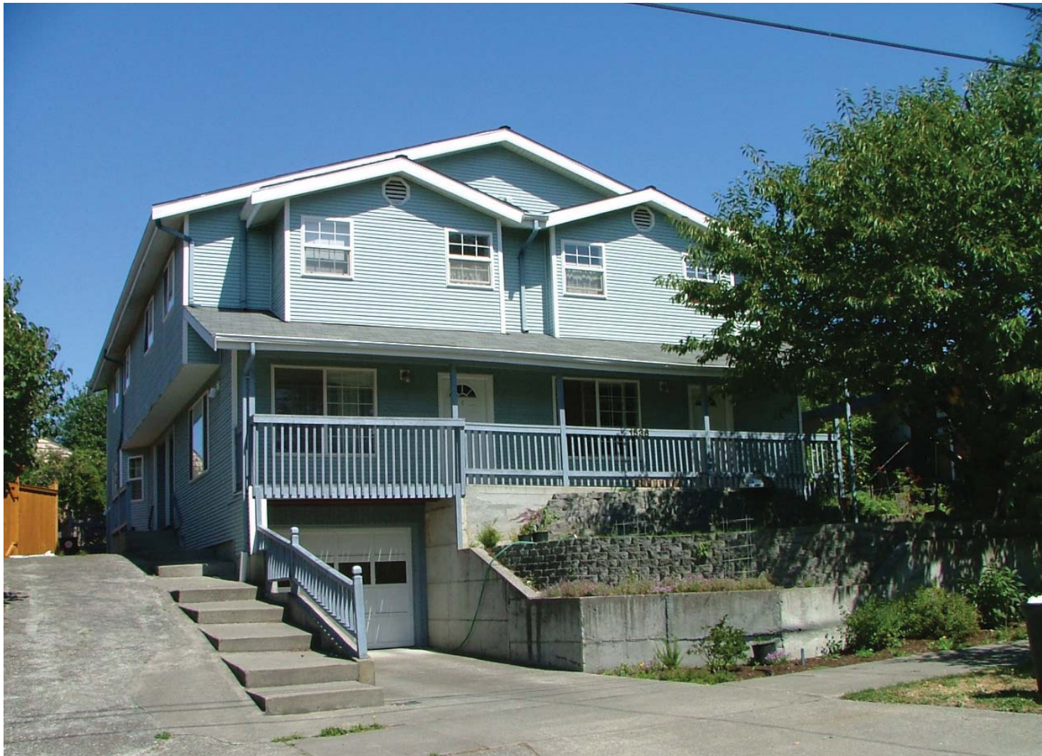
SITE PHOTO: VIEW OF MULTI-FAMILY PROJECT ON NW 62ND AVE WEST OF THE SOUTH
