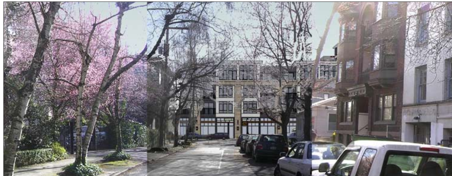
Looking southward on 10th Ave E towards proposed project
