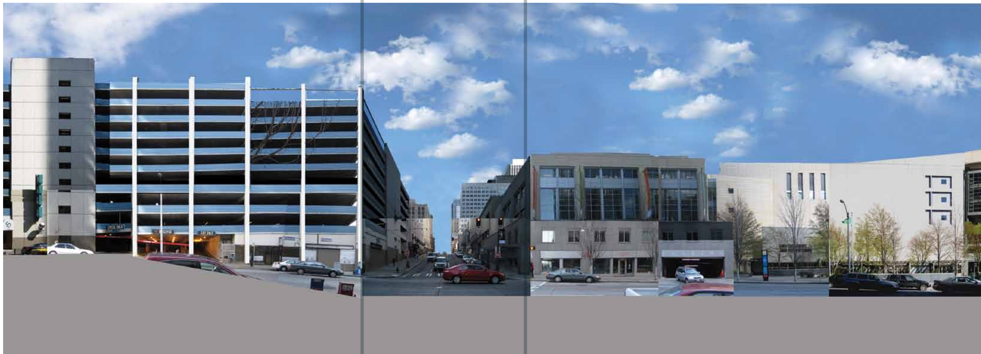
2ND AVENUE ELEVATION FROM SIDEWALK
