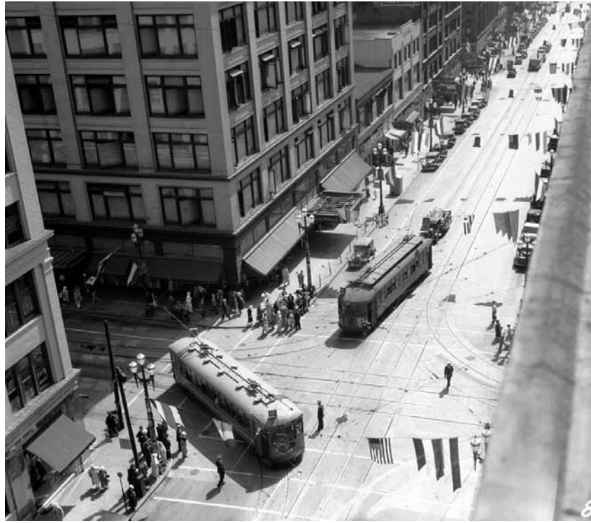
2nd Avenue and Pike St., MacDougall & Southwick Dept. Store, 1934
