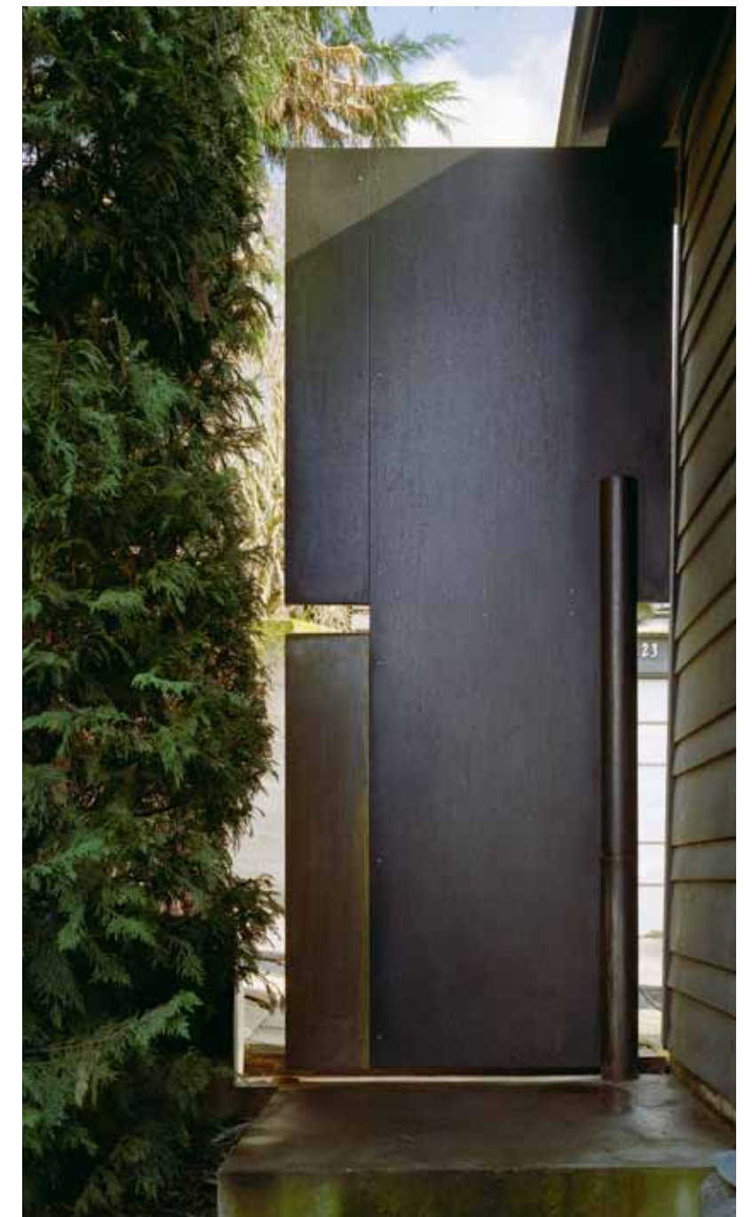
PROMINENT STEEL PIVOT DOOR DETAIL AT BUILDING ENTRY
