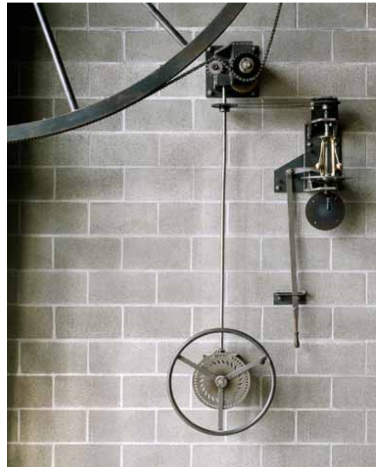
LARGE OPERABLE WINDOW MECHANISM DETAIL
