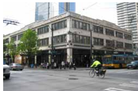
2. KRESS BUILDING (FUTURE IGA GROCERY STORE)
