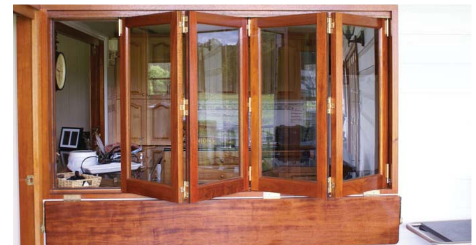
BI-FOLD WINDOWS AT STREET LEVEL AND SECOND FLOOR
