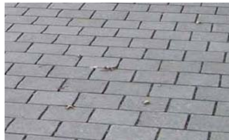
PERVIOUS PAVERS AT PARKING
