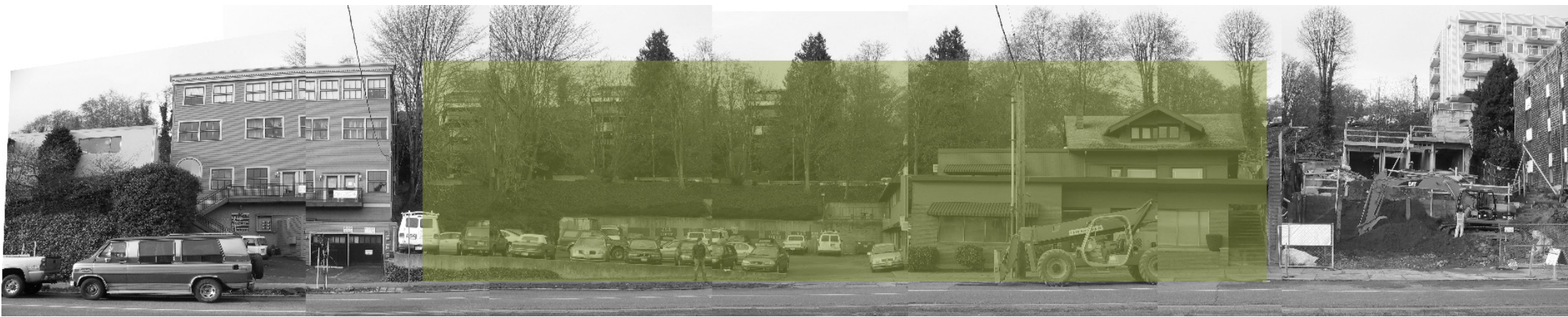
2 VIEW FROM OPPOSITE SIDE OF DEXTER AVE N LOOKING WEST
