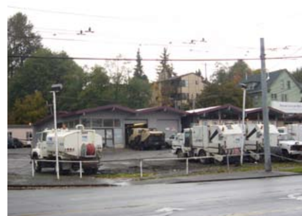
power lines on north portion of site
