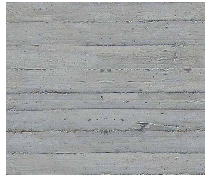
POURED IN PLACE CONCRETE BOARD FORMED TEXTURE
