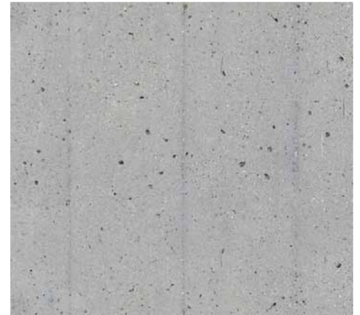
POURED IN PLACE CONCRETE
