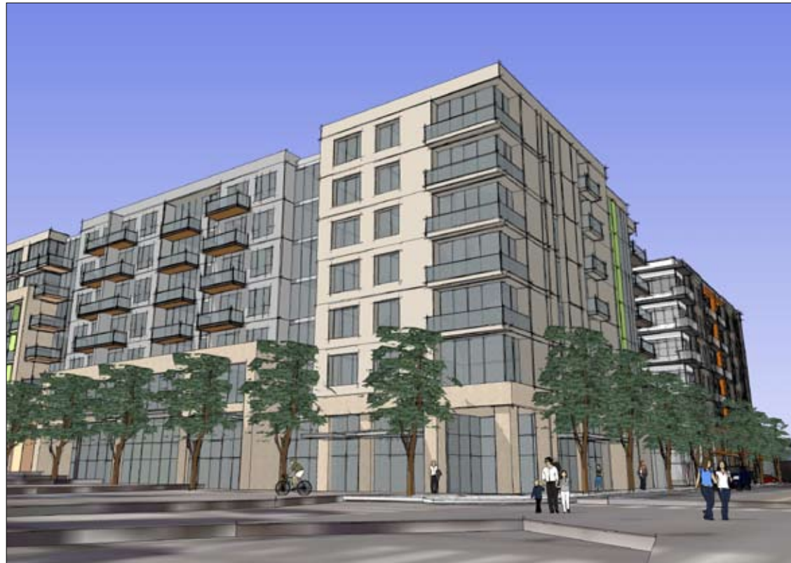
INTERSECTION OF SW ALASKA AND 42ND AVENUE SW
