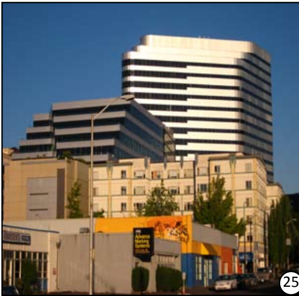
MINOR STREETScape LOOKING EAST Adjacent small businesses, residential, and office towers.
