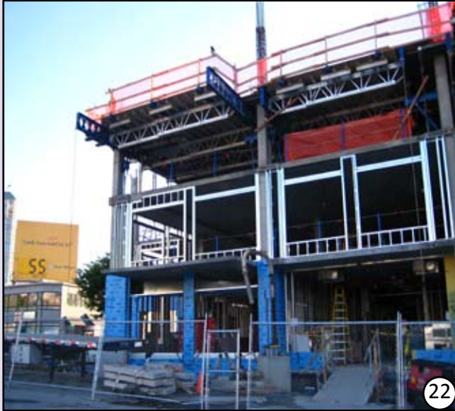
MIRABELLA SENIOR LIVING COMMUNITY Under Construction - High Rise Denny Way and South Lake Union
