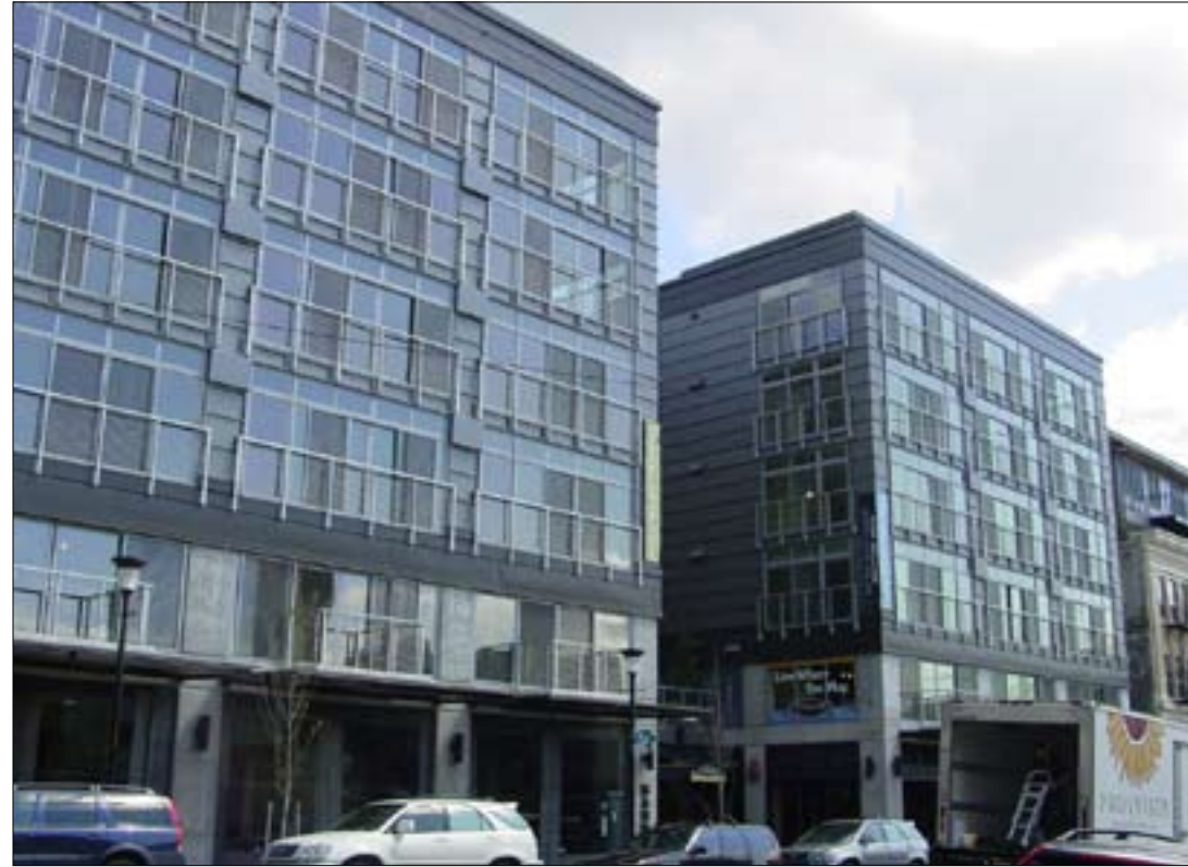
Trace Lofts (12th & Madison) use of metal cladding and architectural concrete at the base
