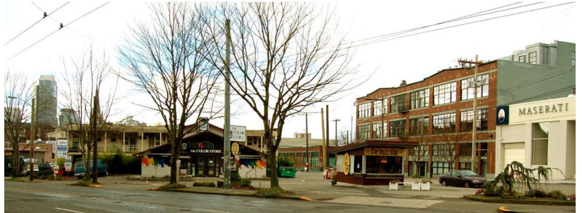
Perspective from East - Existing Buildings on Site & Existing Site Trees
