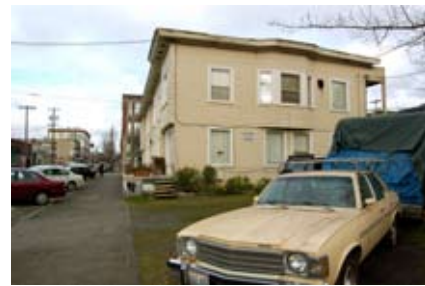
Closeup - Existing Building
