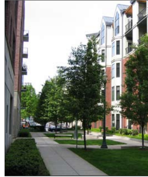
A-7 : Residential Open Space The siting of the building will create usable, attractive, well-integrated open space at street-level as well as upper-levels
