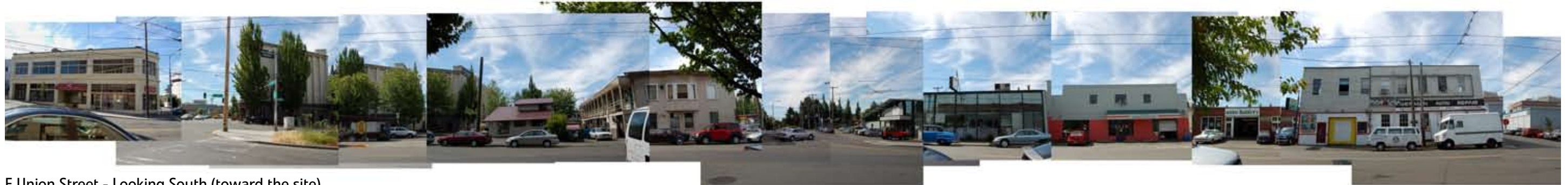
E Union Street - Looking South (toward the site)
