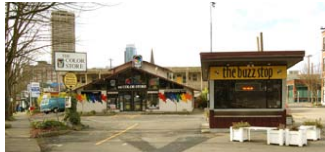
Closeup - Existing Buildings
