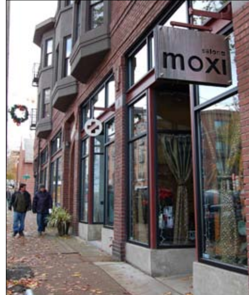
C-3 : Human Scale Incorporate architectural features, elements, and details at a good human scale to create comfortable spaces and invite human activity
