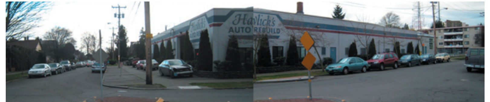
[6] East Olive Street and 22nd Ave looking south west | auto repair
