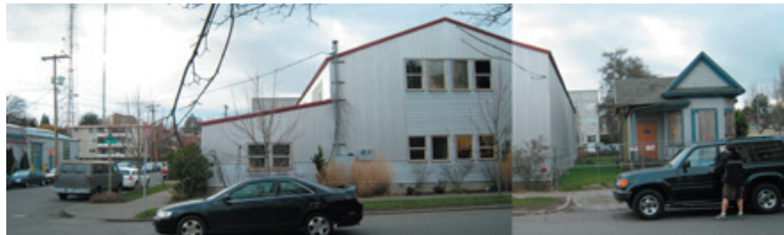
[7] E. Olive St. Looking North | industrial shop & vacant residence
