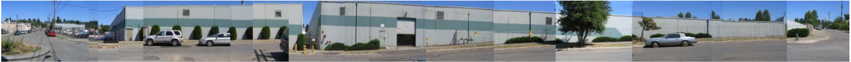
37TH AVENUE S FACING EAST
