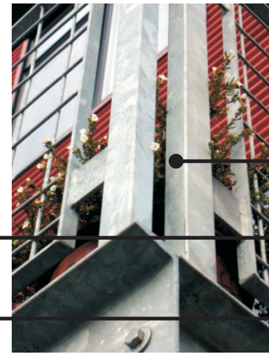
Galvanized Metal Railing and Flashing
