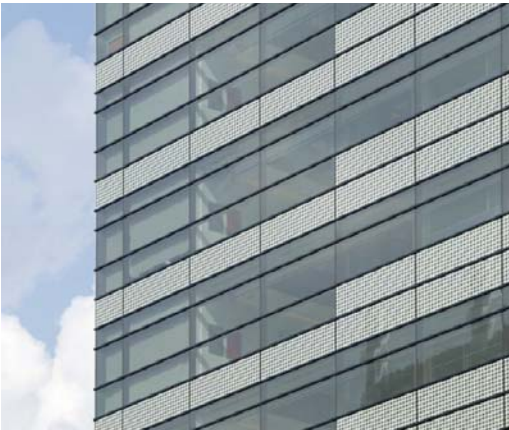
Facade Detail , Leslie L. Dan Pharmacy Building
