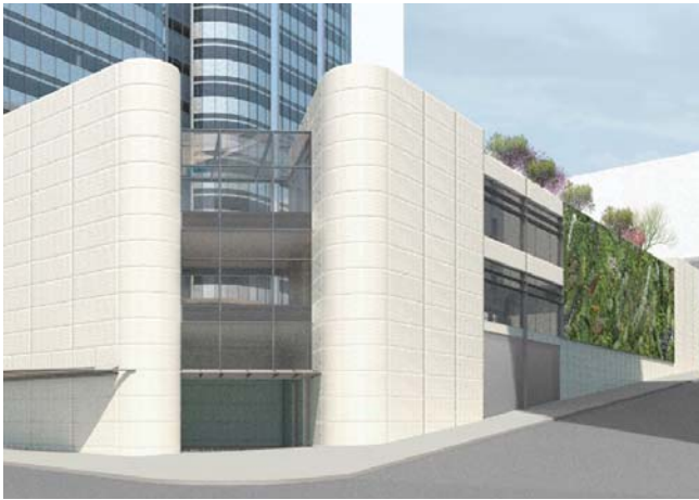
View 1- Corner of Third Avenue and James Street
