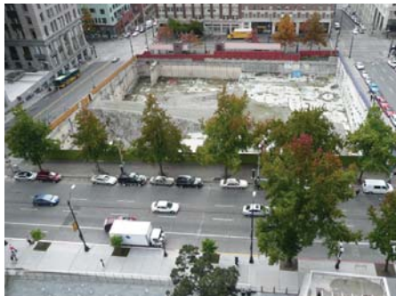
View 6 - Water feature Along Fourth Avenue
