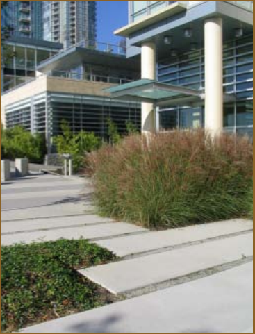
Integrally Colored CIP Concrete
