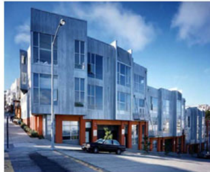
18TH + ARKANSAS, SAN FRANCISCO, CALIFORNIA DAVID BAKER + PARTNERS ARCHITECTS
