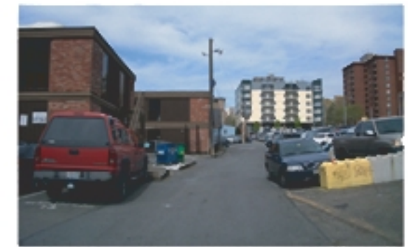
5. Alley North of Property - Looking North
