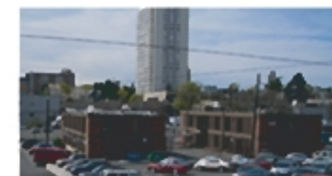
9. 2 Story office buildings
