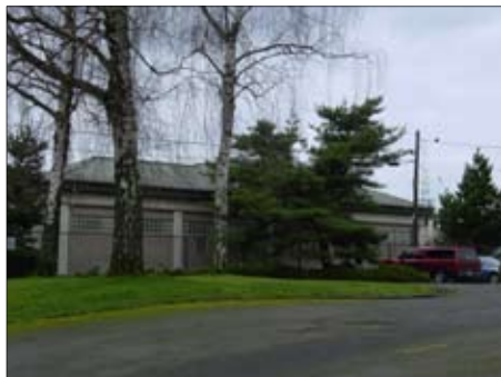
(C) Reservoir Building
