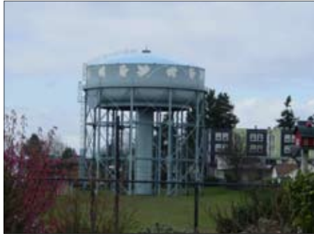
(A) Water Tower
