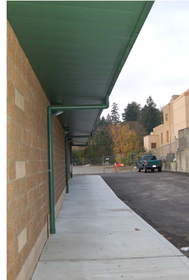
EXISTING OVERHANG @ RETAIL
