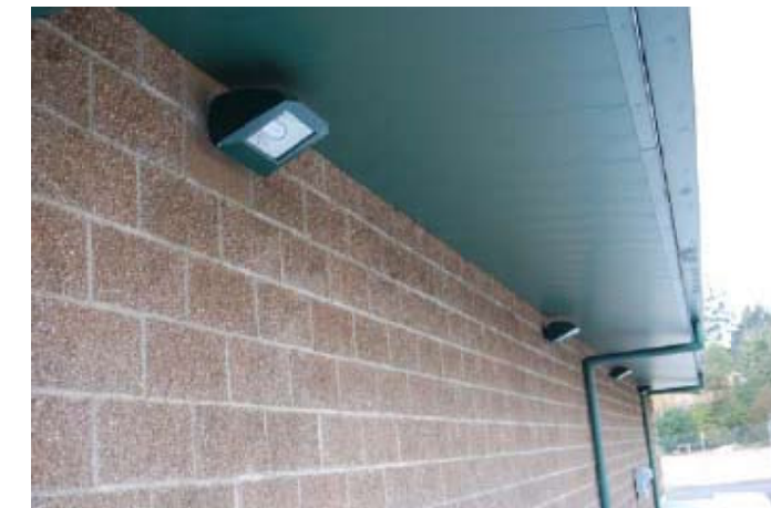
EXISTING WALL PACK FIXTURES
