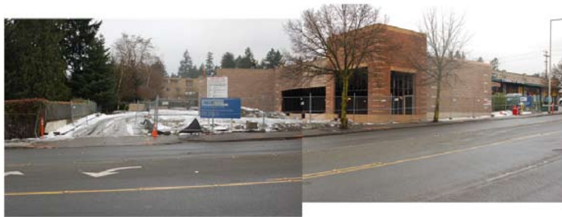
VIEW OF SITE FROM 15TH AVENUE NE LOOKING WEST
