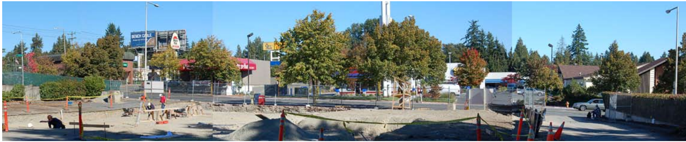
VIEW FROM SITE LOOKING EAST TOWARDS 15TH AVE NE
