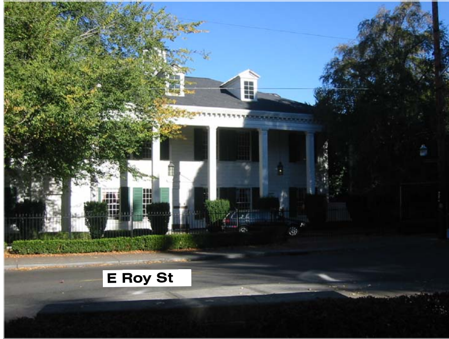
View of multifamily in L3 zone along E Roy Street.
