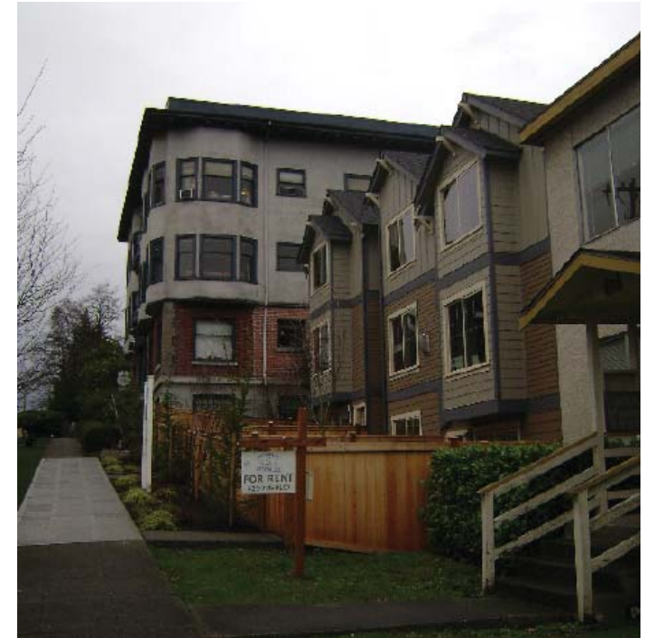
New Townhouses & Existing Multifamily Looking N. on 11th
