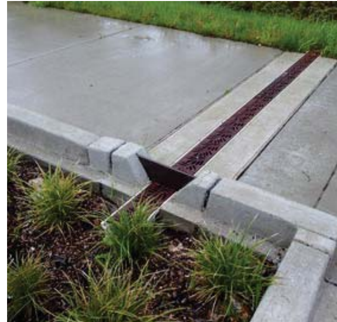
above: diagram illustrating drainage of view corridor green roof below: images of conveyance across sidewalk to rain gardens / weirs
