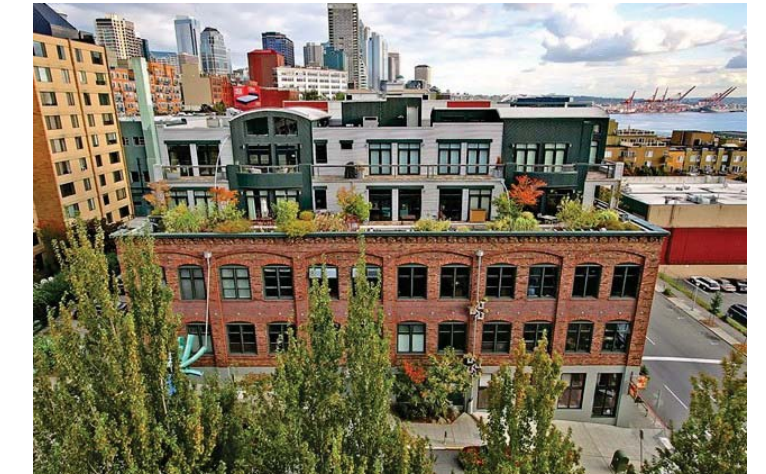
81 Vine Street (renovation / addition)
