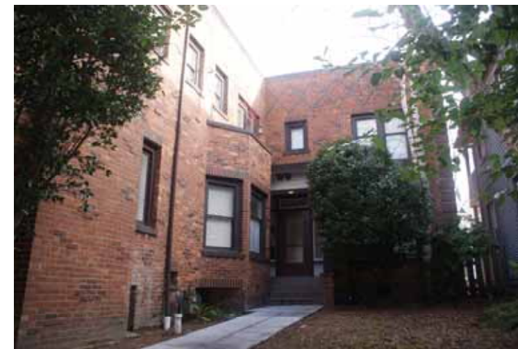
Belmont Ave—view of courtyard of building north of project
