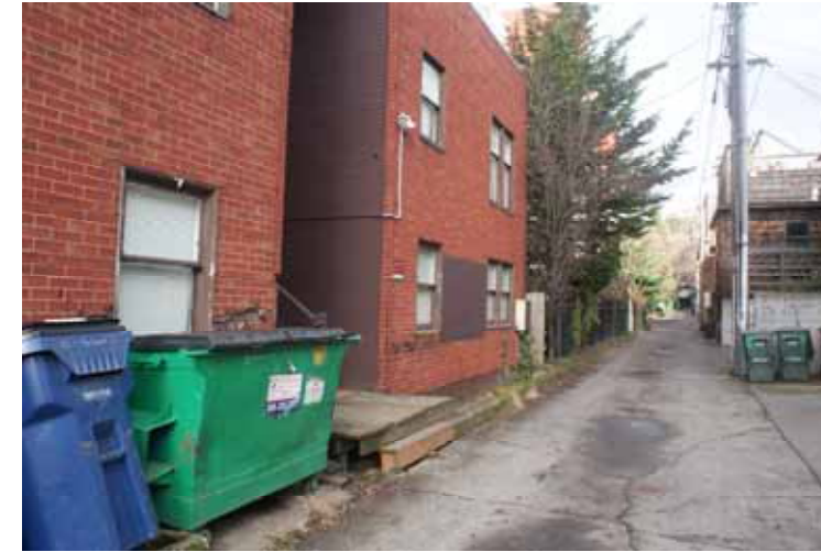
Alley—existing buildings to be demolished
