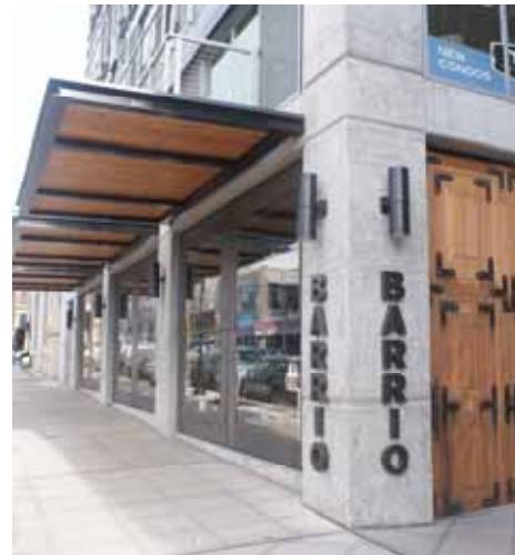
Trace Lofts— “Heavy” Base
