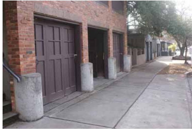
Belmont Ave—West sidewalk looking south
