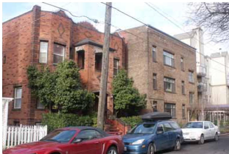
Belmont Ave—East side of street
