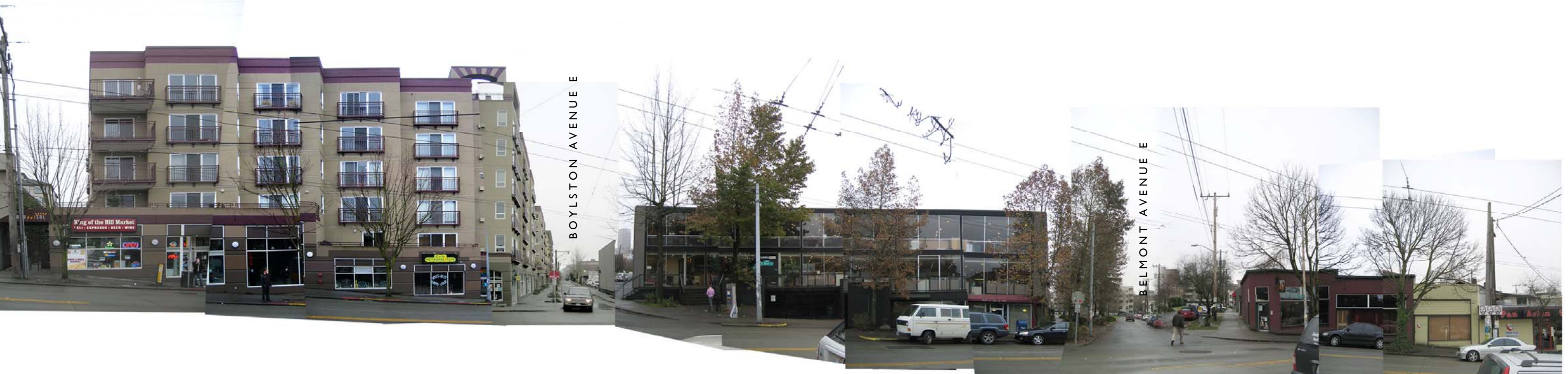
E OLIVE WAY LOOKING SOUTH
