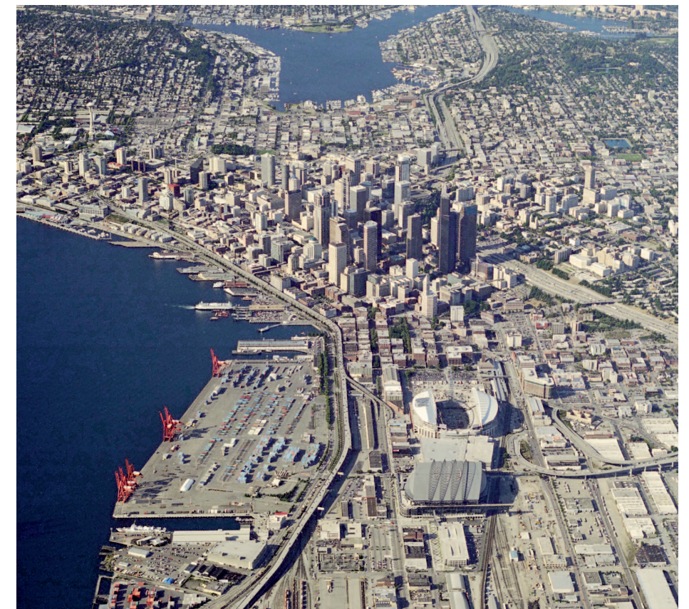
Figure 3: Overview of Seattle, looking north along Viaduct
