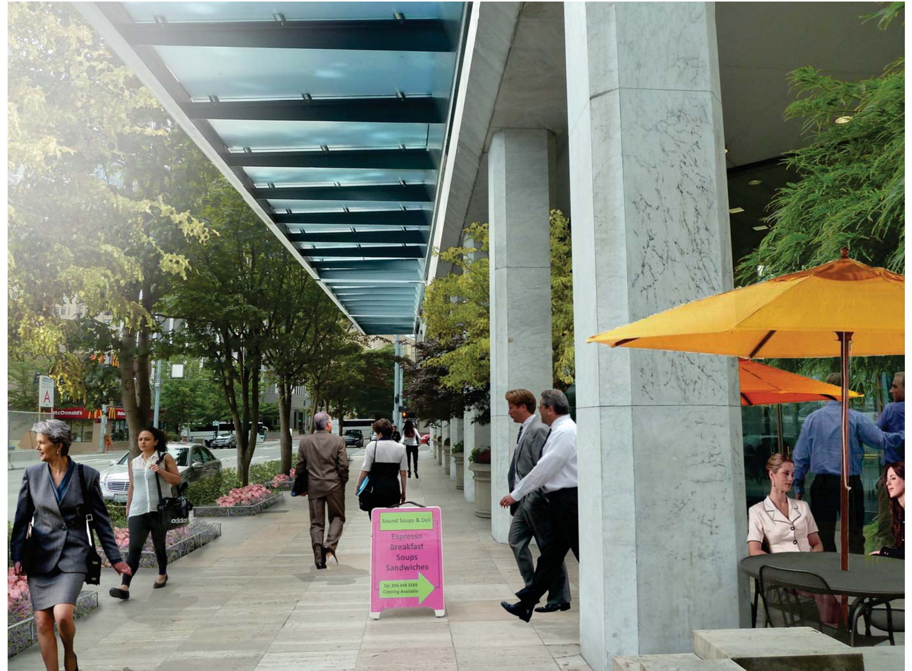
Architectural Canopy Along 6th Avenue & Virginia
