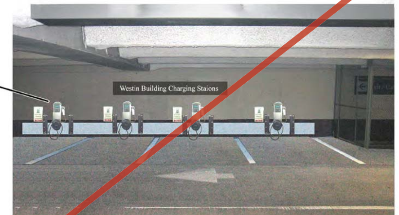
(B) CHARGING STATIONS
